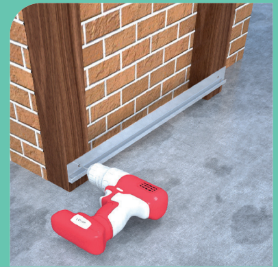
3) Install starter bar, ensuring that it is at least 30mm from the ground.
